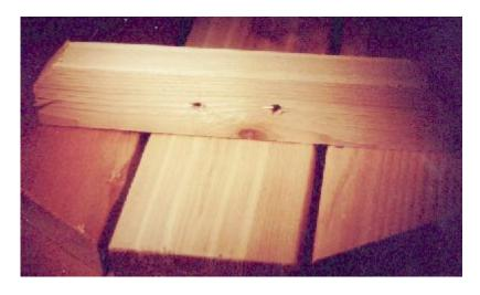
23) SCREW DOWN THE 13 1/2" PIECES USING THE 3" PLATED DECK SCREWS. SCREW 2 SCREWS PER BOARD. COUNTER SINK THE SCREWS ABOUT 1/4" TO SECURE IT GOOD TO THE TABLE TOP.
